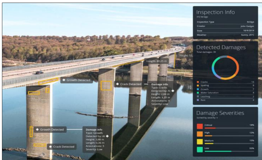
Fig 3. Bridge Inspection Using AI Integ Digital Twin Platform
