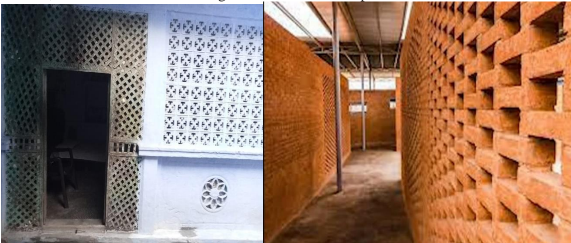
Figure 5,6 – Traditional Jallies In Vernacular Based Architecture In Houses
