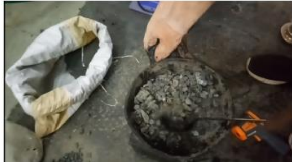
Fig. 4. Mixing of aggregates with bitumen
