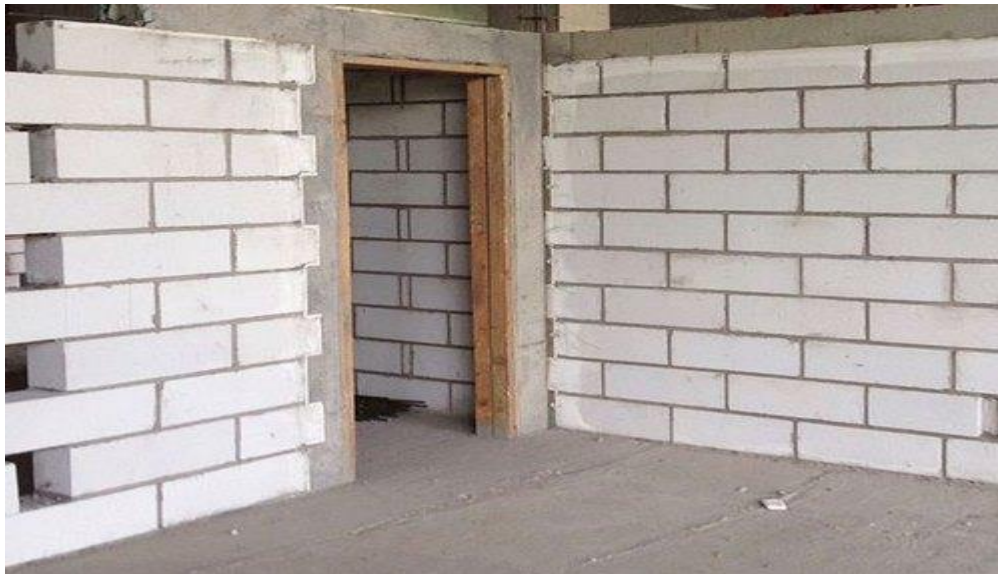
Figure 6: Application of AAC blocks
