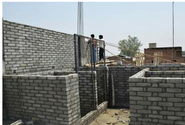
Figure 4: Fly ash brick and its application
